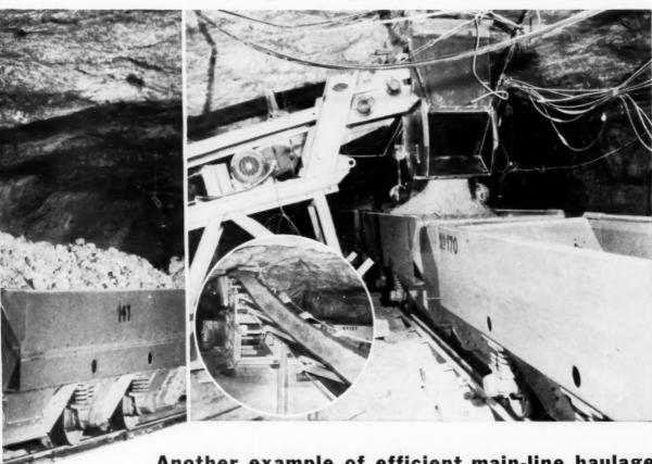
Another example of efficient main-line haulage with S-D "Automatic" Bottom Dumping Mine Cars!
